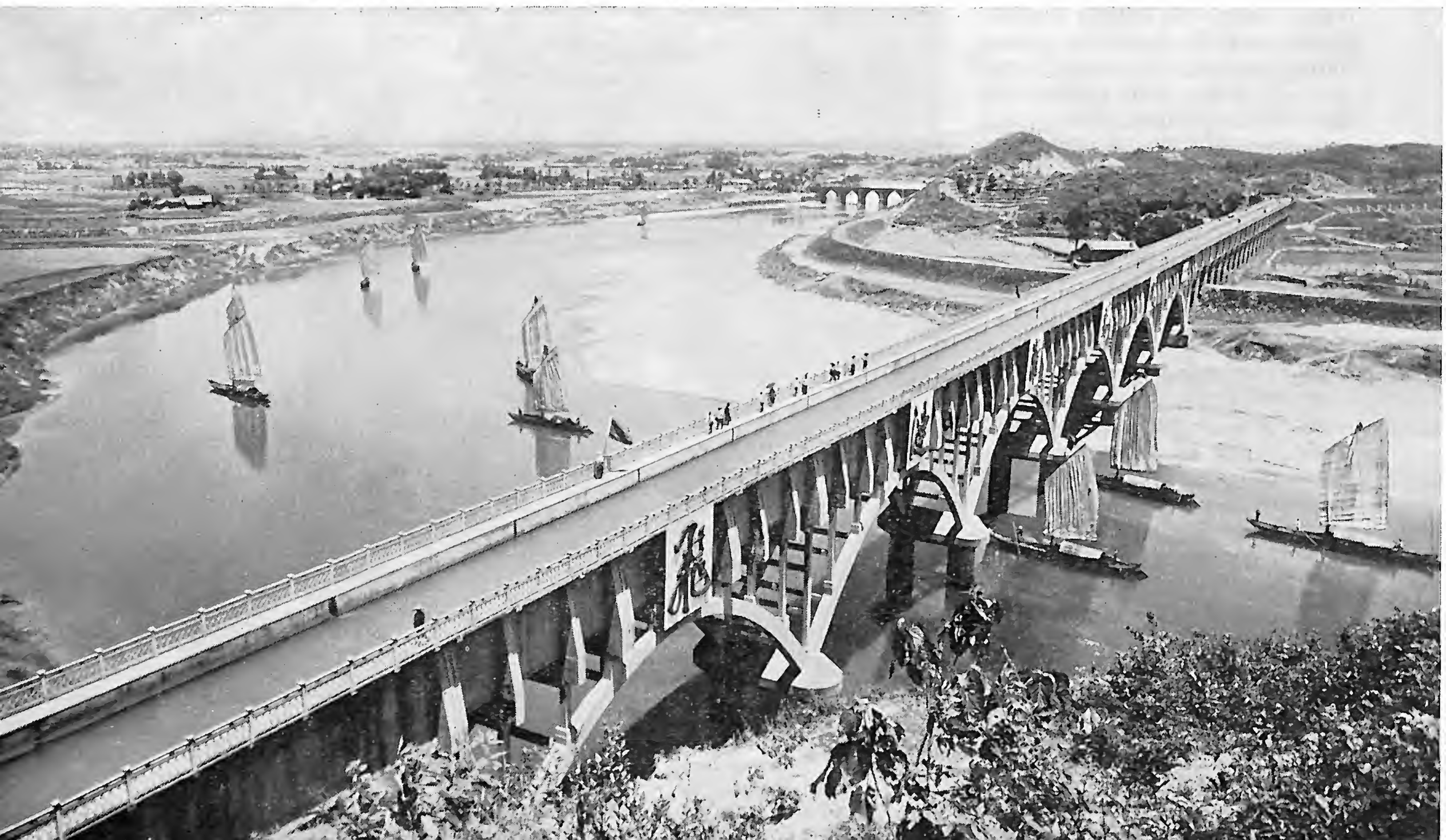
An aqueduct on the northern trunk canal of the huge Shaoshan irrigation system, the first such to be built in Hunan province.
